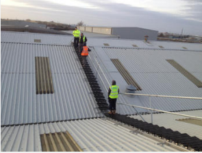
Total Collective Protection on a Cladded Roof
