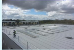
Total Collective Protection on a Cladded Roof
